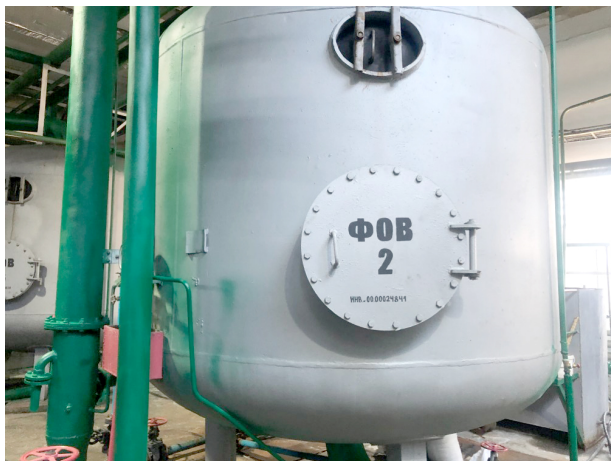
Рис. 1. Установка ФОВ Fig. 1. Installation of the water purification filter
