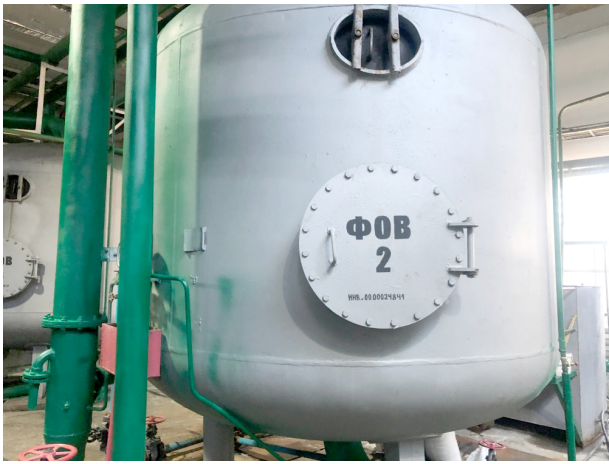
Рис. 1. Установка ФОВ Fig. 1. Installation of the water purification filter
